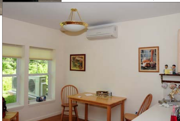
The one-bedroom units at the affordable housing community for people with special needs are heated and cooled by 18K Btu/h Daikin outdoor units.
